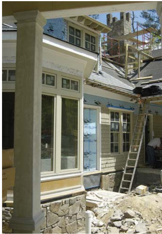
Attention to the details: Above, exterior finishes protects the integrity of the structural components, such as the Delta® Dry drainage plane that gets covered up by the external cladding.
